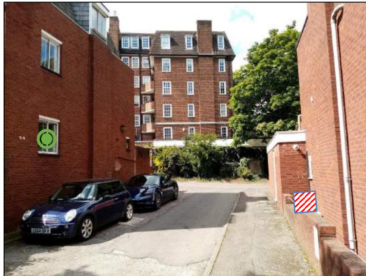
Figure 2.3 Identified receiver and proposed plant unit installation
